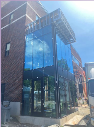
Main Office Renovation
